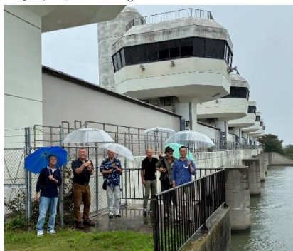
坊僧川津波水門
